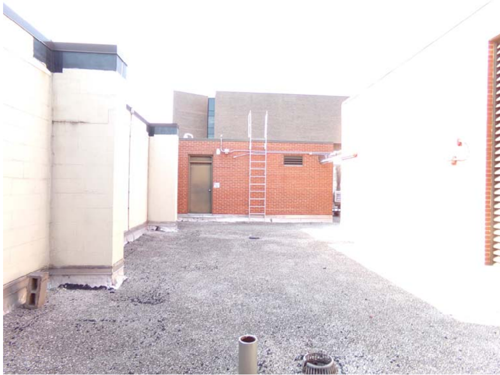
Pharmacy Roof A-East side, looking South
