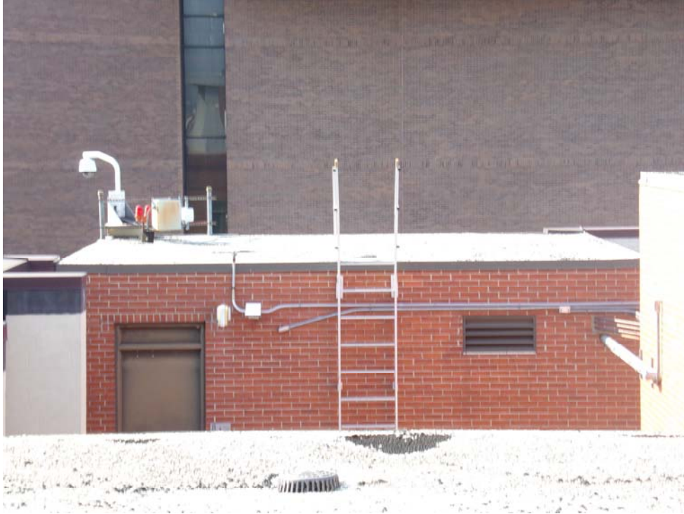
Pharmacy Roof E-Looking South
