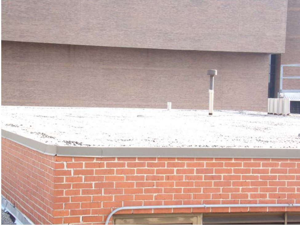
Pharmacy Roof G-LookingSouth
