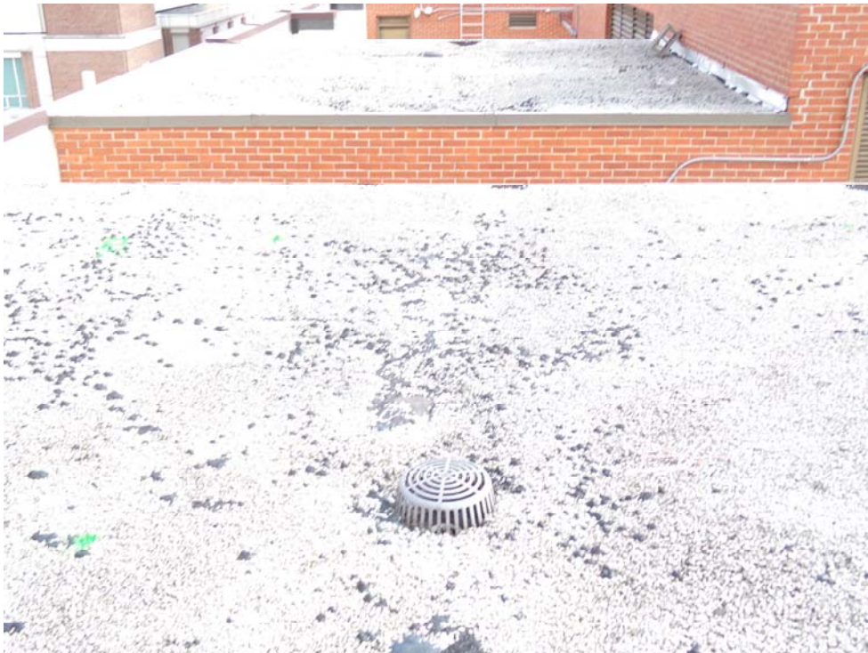
Pharmacy Roof B-Looking South
