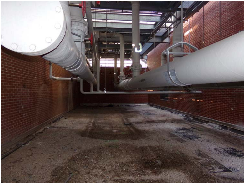
Pharmacy Roof H-Looking South
