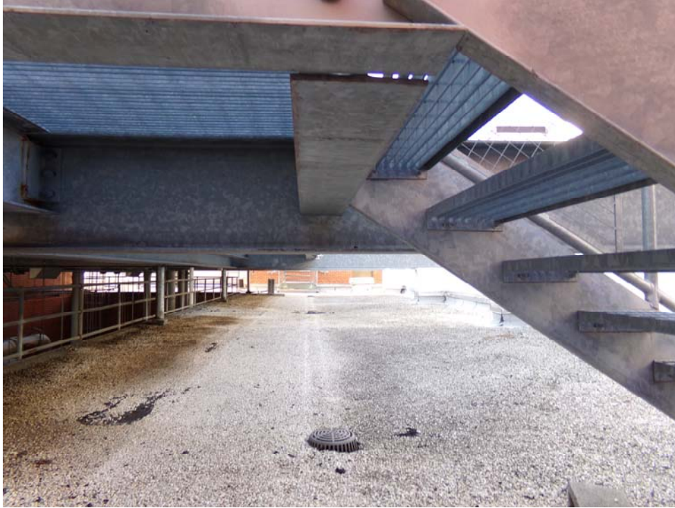
Pharmacy Roof A-West side, looking South
