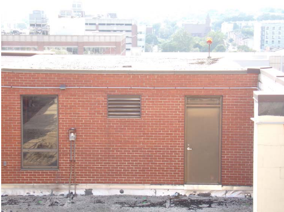
Pharmacy Roof D-Looking South
