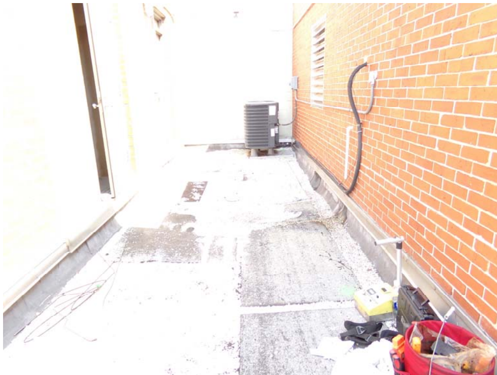
Pharmacy Roof A-East neck, looking East
